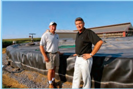
Luke Brubaker's Methane Digester
